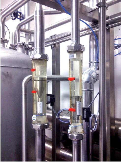
Monitoring of the flow of concentrate and recirculation of a Reverse Osmosis Water Treatment Plant
