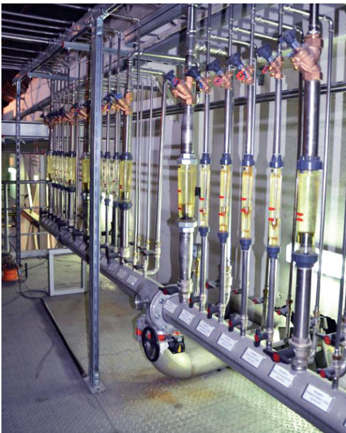
Cooling Water Distribution System in a Glass Melting Factory
