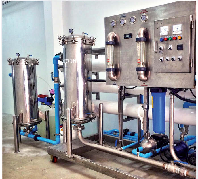
Reverse Osmosis System
